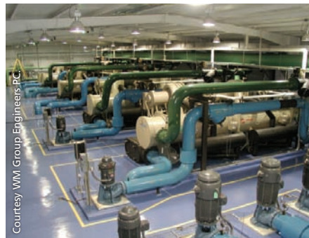
These images from a chilled-water plant at a major university show the plant before and after numerous pumps were removed.
